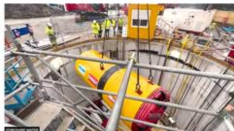
A remote-controlled tunnelling machine is being used to lay a new 3000 (2,624ft) sewer under the A63 in Ilkley
